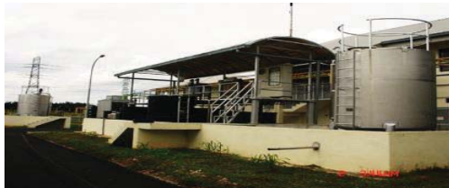
Figure 5. Water treatment plant [5]
